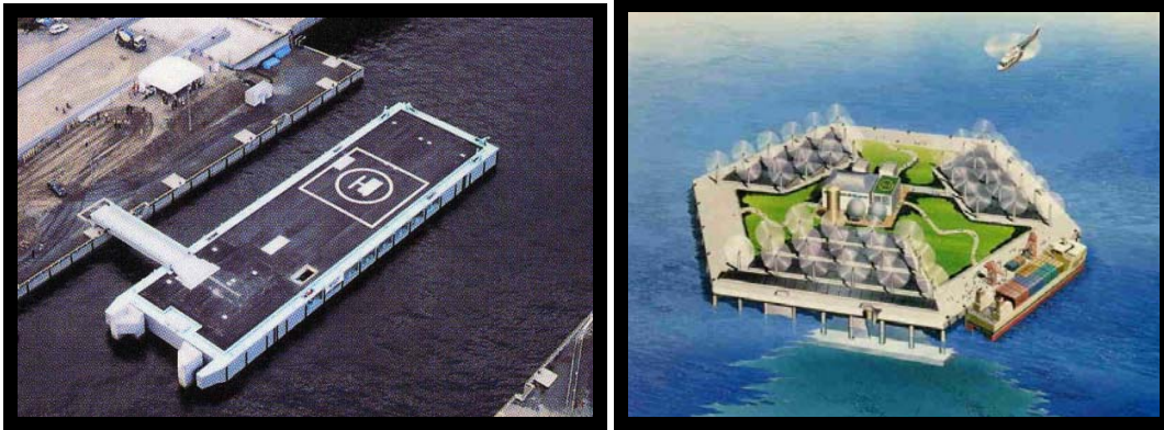
Figure 2. Emergency mobile unit in Tokyo gulf (left). Prototype for installation of offshore wind farm in open sea (right)
