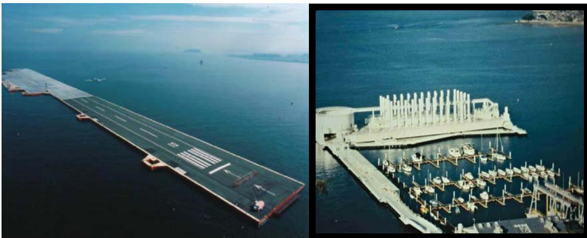
Figure 1. Floating airport (left). Floating island with touristic & recreational support installations (right) in Onomichi, Hiroshima, Japan.
